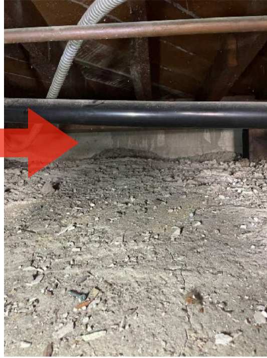
Item Image 2 - Crawlspace
