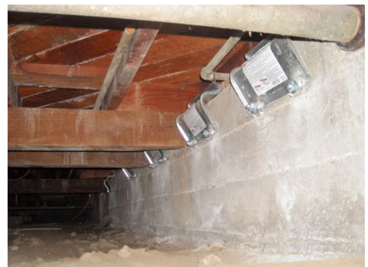
No Cripple Wall Example - UFP only
