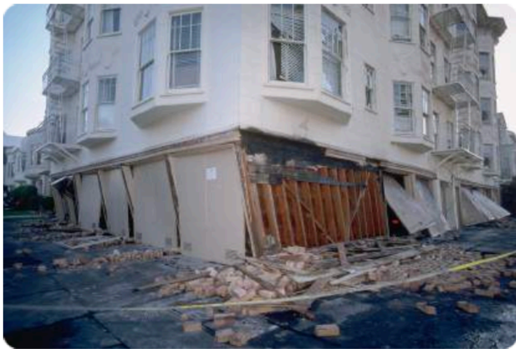
Apartment Bldg Failure
